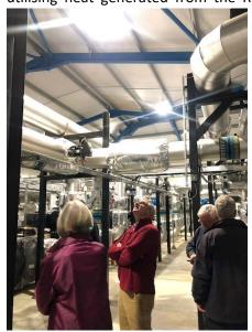
process involves extraction of river water (heated by the sun) which is passed through a heat exchanger and is then discharged straight back into the river having removed a couple of
